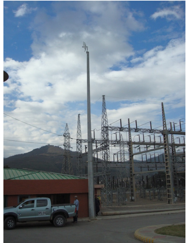
Figure 6. EBSA Building No. 1
