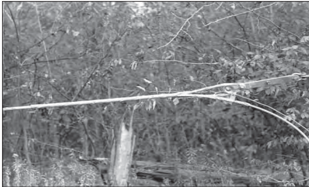
FIBERLIGN Formed Wire Dead-end Installed
