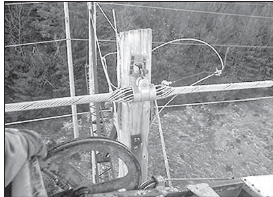
SINGLE FIBERLIGN SUSPENSION FOR OPTICAL GROUND WIRE (OPGW)
